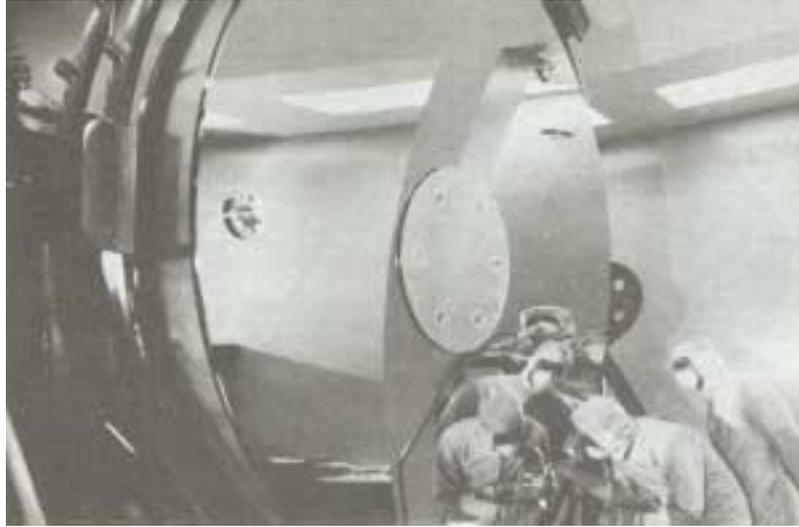
**Figure 2.** The HST primary mirror at Perkin Elmers, with two of the three pads clearly visible in the mirror .
