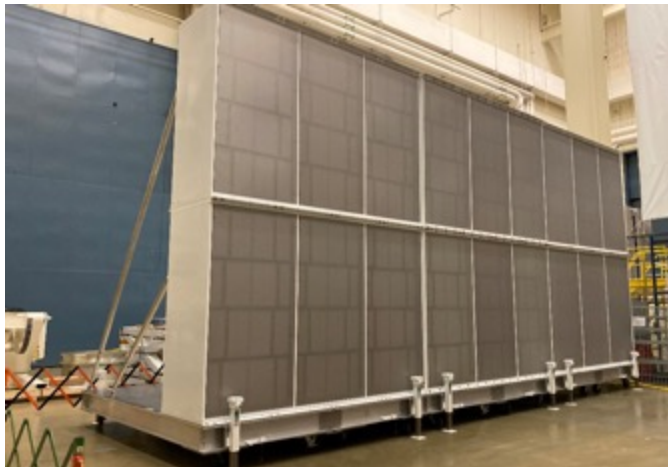
One side of HEPA filter wall (3 dollies 2 HEPA units per dolly)
